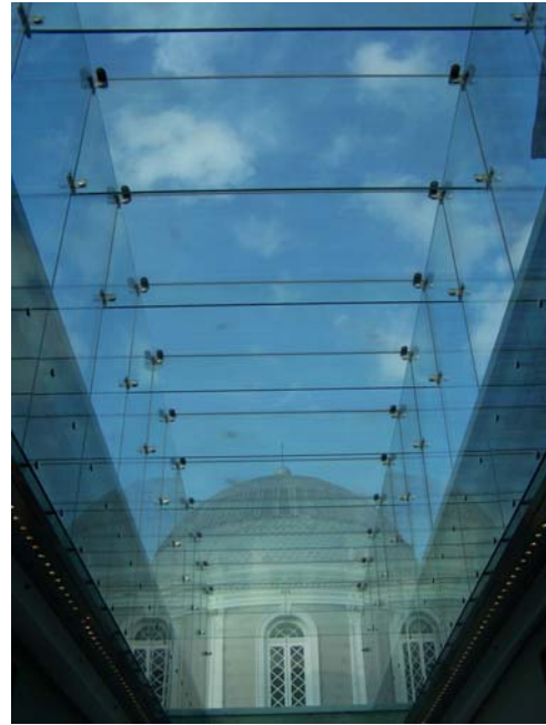
Figure 3. View of Dome from inside the Glass Passage
